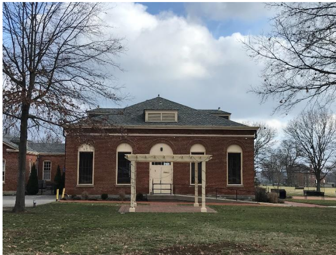
Mess Hall Pergola
